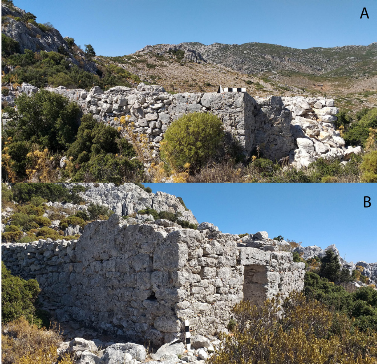
Figure 23. View from northern wall of apsidal structure (A); gate lento with a closer image of masonry (B), Korsan Kale, Söğüt.
